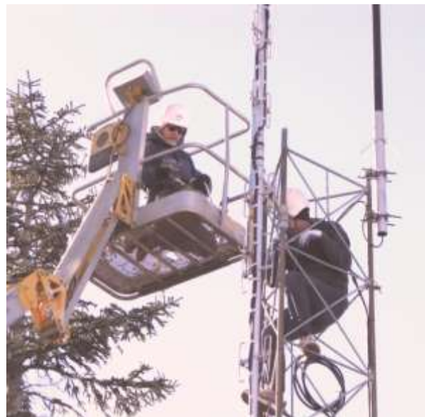
Jim Campbell, N7QME and Marc Peterson, W7PM removing broken 4 bay antenna from South Saddle tower
