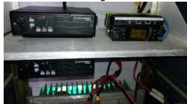
Left: Shown on top is the ARCOM 210. With the 147.320 Quantar shown on top. This is connected to Port 1 on the Arcom. The gold box is the 442.325 UHF duplexer and below that, is the 442.325 Quantar. Both repeaters are set for 60 watts out, with about 305 watts out the duplexers to the antennas, with zero reflected when running properly.
